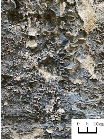
Figure 7. The surface of stone relics affected by lichen and moss (Nankan Bas-reliefs, Bazhong, Sichuan, China) ©
